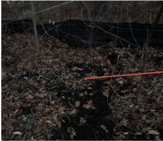
Photo 9: Sediment fence at tree line by 14 th hole is allowing flow underneath in one location and should be repaired. An additional stone check dam could be added upgradient of protected area to disrupt channelized flows.
