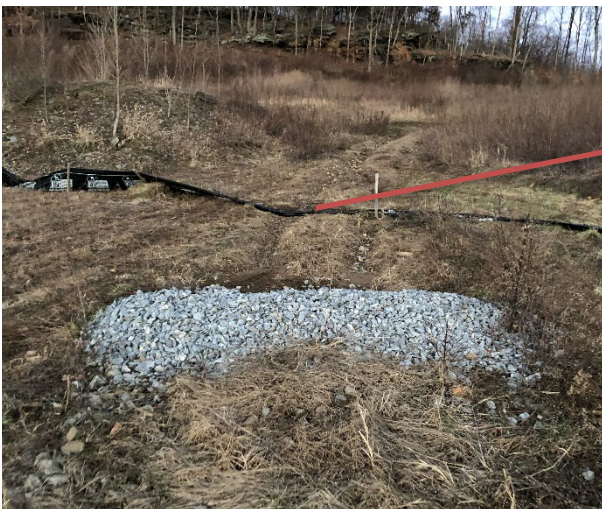
Photo 8: Sediment fence row across 11 th hole tee box area has been knocked over by ATV traffic.
