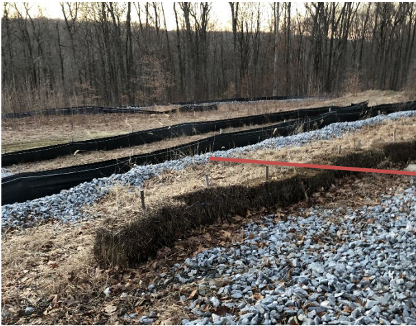
Photo 3: Some sediment fence repairs are needed for undermining at upper and lower sediment fence rows. Intermediate sediment fence through sapling stand is beginning to fail and should be restaked. Sediment should be removed from check dams.
