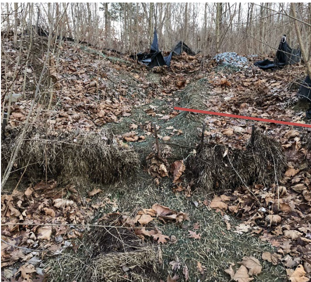
Photo 4: Staked hay bales and sediment fence in area shown have failed/deteriorated. There is erosion under the erosion control mat. Check dams should be added to replace deteriorated erosion control measures.
