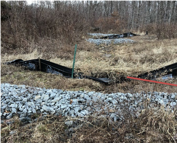
Photo 7: Stone check dams across the 7 th hole fairway hillside remain in good condition. Sediment fence rows and hay bales have deteriorated. Since upgradient areas are vegetated the sediment fence could be replaced with additional stone check dams to prevent erosion from channelized flows..
