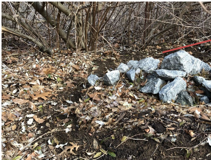
Photo 2: Stone check dam in path leading to water crossing has reached capacity and allowed sediment to flow around check dam.
