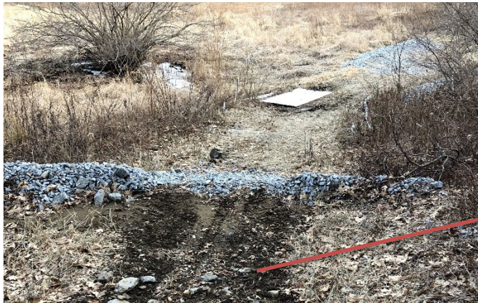
Photo 1: Stone check dam immediately upgradient of main entry water crossing has flattened due to A1V traffic and has reached capacity with collected sediment.
