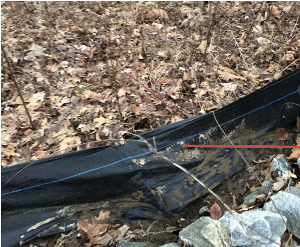
Photo 5: Stone check dams and staked hay bales are in good condition. Collected sediment should be removed and sediment fence repaired.
