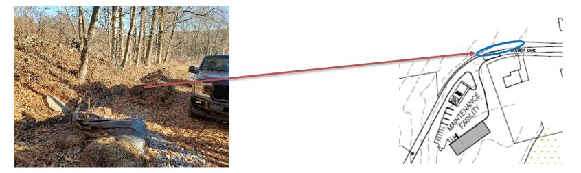
Photo 6: Staked hay bales and sediment fence at construction entrance have deteriorated and been removed since last inspection.
