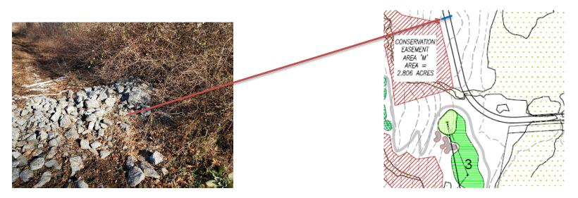
Photo 2: Stone check dam in path leading to water crossing has reached capacity and allowed sediment to flow around check dam.
