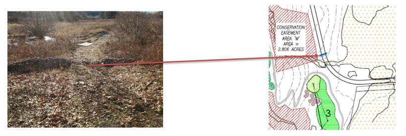
Photo 1: Stone check dam immediately upgradient of main entry water crossing has flatten due to ATV traffic and has reached capacity with collected sediment.
