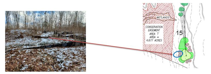
Photo 4: Staked hay bales and sediment fence in area shown have failed/deteriorated. Stone check dam downgradient remains in good condition with ample storage capacity available.
