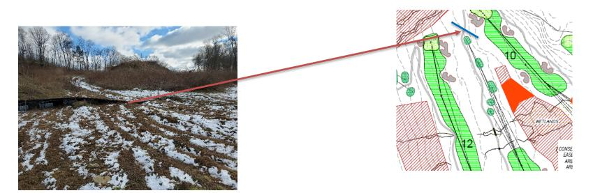
Photo 8: Sediment fence row across 11<sup>th</sup> hole tee box area has been knocked over by ATV traffic but area was stable at time of inspection.
