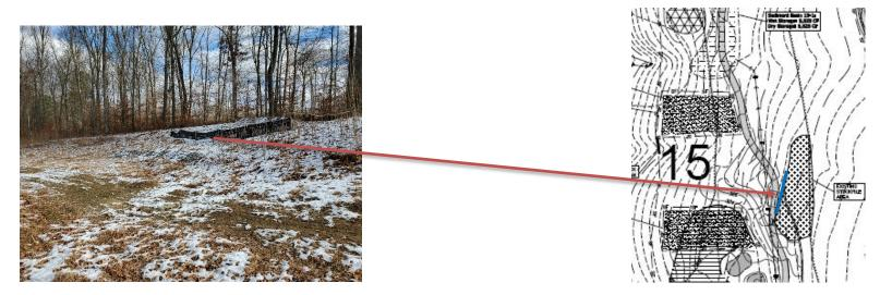
Photo 5: Stone check dams, staked hay bales, and sediment fence remain in good condition with ample storage capacity available.
