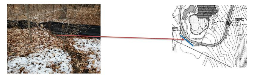
Photo 9: Sediment fence at tree line by 14<sup>th</sup> hole is allowing flow underneath in one location and needs to be repaired.
