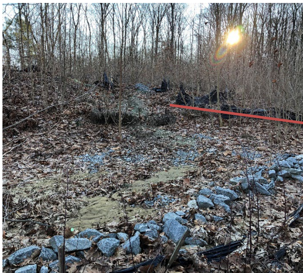
Photo 4: Staked hay bales and sediment fence in area shown have failed/deteriorated. There is erosion under the erosion control mat. Check dams should be added to replace deteriorated erosion control measures. Collected sediment should be removed.
