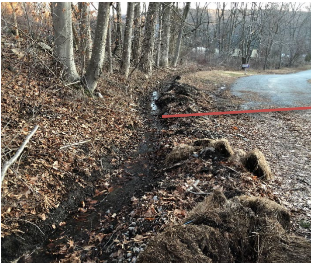
Photo 6: Recently constructed swale carrying flow to downgradient drainage structure. No signs of erosion in swale.
