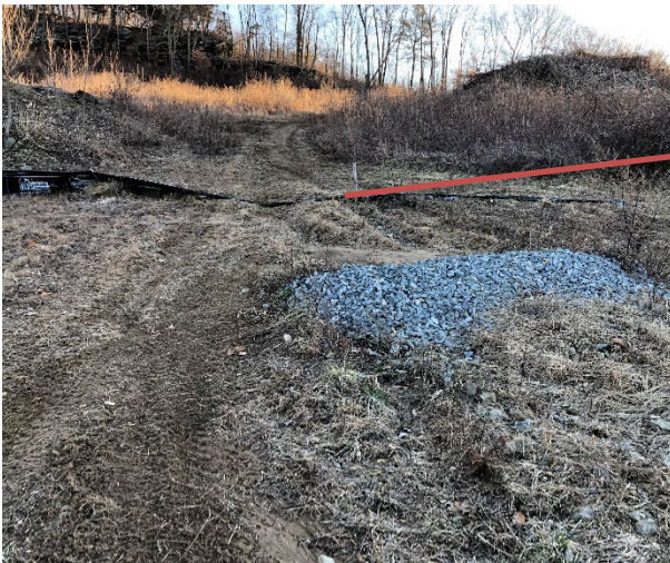
Photo 8: Sediment fence row across 11 th hole tee box area has been knocked over by ATV traffic. Remove collected sediment from check dam.
