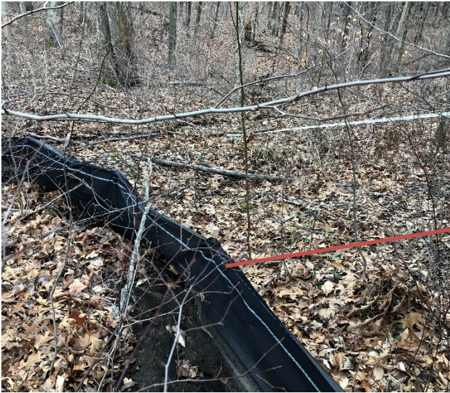
Photo 9: Sediment fence at tree line by 14 th hole is allowing flow underneath in two location and should be repaired and reinforced with a stone check dam. An additional stone check dam could be added upgradient of protected area to disrupt channelized flows.
