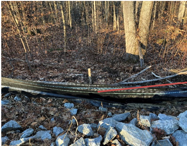
Photo 3: Some sediment fence repairs are needed for undermining at upper and lower sediment fence rows. Undermined areas should be reinforced with stone check dams. Intermediate sediment fence through sapling stand is beginning to fail and should be re-staked. Sediment should be removed from check dams.
