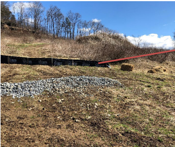
Photo 8: Sediment fence row across 11 th hole tee box area has been repaired and stone check dam upgraded. A hay bale check dam has been added upgradient of the sediment fence. All measures are in good condition, some off-road vehicle traffic has damaged a portion of the hay bale check dam but adequate storage capacity is still available.
