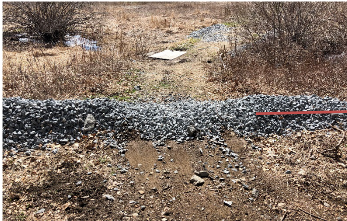
Photo 1: Stone check dam immediately upgradient of main entry water crossing is in good condition. Some off-road vehicles have started to damage the check dams, but ample capacity is still available.
