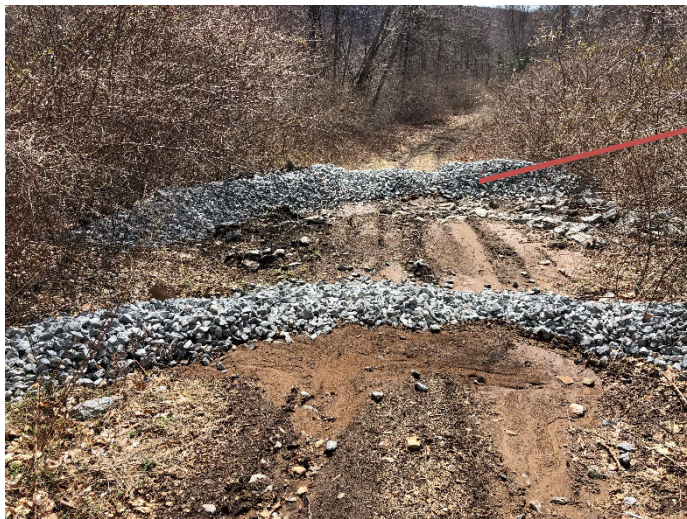
Photo 2: Stone check dams in path leading to water crossing are in good condition. Some off-road vehicles have started to damage the check dams, but ample capacity is still available.
