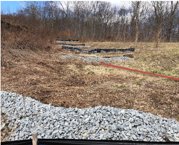
Photo 7: Stone check dams and sediment fence across the 7 th hole fairway hillside are in good condition, filtered flow observed.
