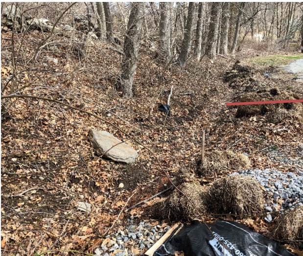
Photo 6 : No signs of erosion in swale at entrance driveway.
