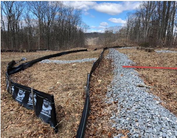
Photo 3: Sediment fence has been repaired and reinforced with stone check dams and is in good condition.
