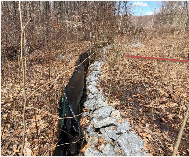
Photo 5 : Filtered flow along 15 th fairway at stone check dams and perimeter sediment fence.
