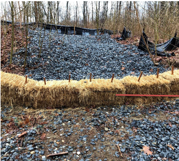
Photo 4: Staked hay bales have been replaced and eroded area has been stabilized with stone and is in good condition.
