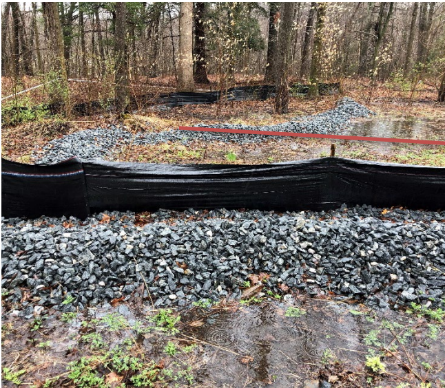
Photo 9: Sediment fence has been repaired and additional stone check dams added to disrupt flows. Measures are in good condition and flow is filtered by stone check dams.
