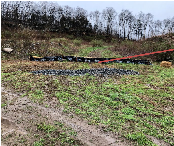
Photo 8: Sediment fence row across 11 th hole tee box area has been repaired and stone check dam upgraded. A hay bale check dam has been added upgradient of the sediment fence. All measures are in good condition, some off-road vehicle traffic has damaged a portion of the hay bale check dam but adequate storage capacity is still available.
