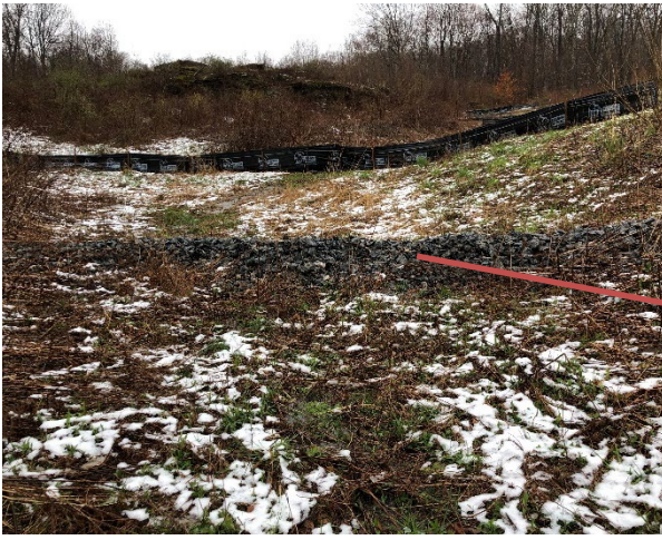
Photo 7: Stone check dams across the 7 th hole fairway hillside are in good condition, filtered flow observed.
