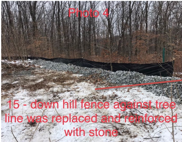
Photo 3: Sediment fence has been repaired and reinforced with stone check dams.
