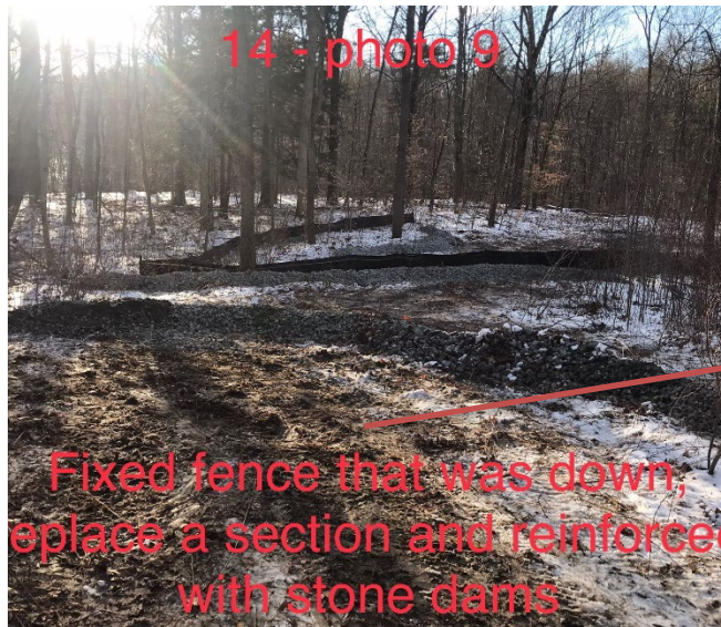
Photo 9 : Sediment fence has been repaired and additional stone check dams added to disrupt flows.
