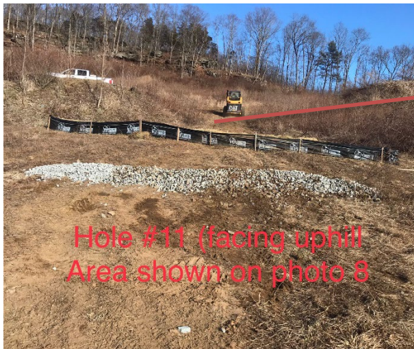
Photo 8: Sediment fence row across 11 th hole tee box area has been repaired and stone check dam upgraded. A hay bale check dam has been added upgradient of the sediment fence.
