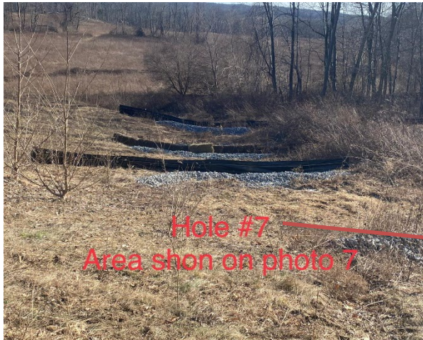
Photo 7: Stone check dams across the 7 th hole fairway hillside remain in good condition. Sediment fence rows and hay bales have been repaired and reinforced with stone check dams.
