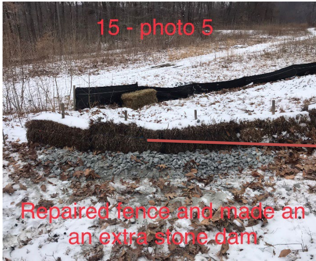
Photo 5: Stone check dams and staked hay bales are in good condition. Sediment fence has been repaired and an additional stone check dam has been added.
