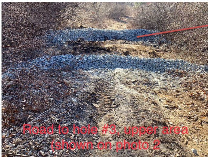
Photo 2: Stone check dam in path leading to water crossing has been repaired and an additional check dam has been added.
