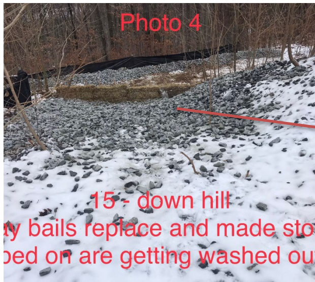
Photo 4: Staked hay bales have been replaced and eroded area has been stabilized with stone.
